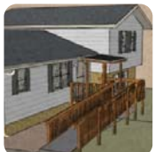
(b) wheelchair ramp
